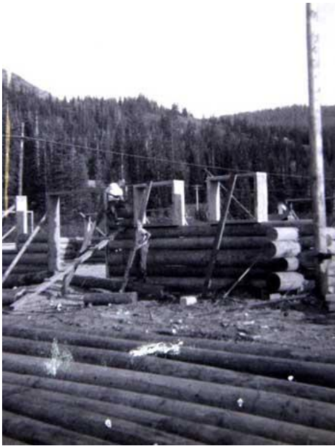
Building the "Bowery", today's Brighton Village Store.
