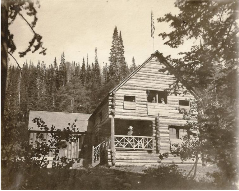
Balsam Hill Cabin 1901, with its "most artistic railing" made of aspen and the little framed cabin attached, becoming the kitchen
