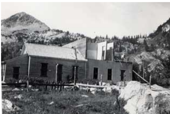
The Brighton Hotel just before and during demolition. 1945 Photos courtesy of Adrienne Aldous and the Moyle Family Collection
